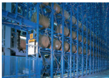
Automatic warehouses for paper rolls
